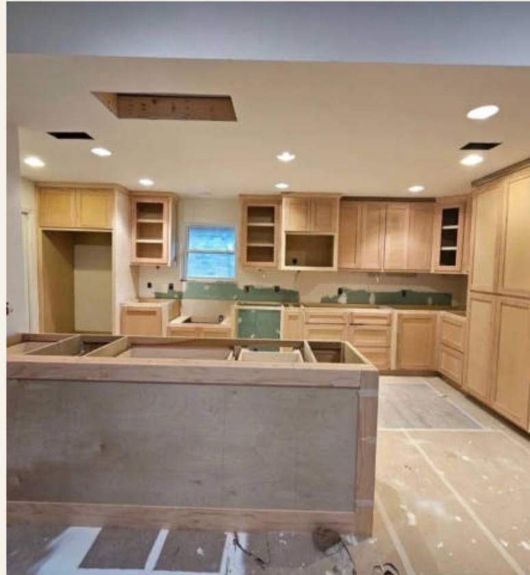
Island and perimeter cabinetry before final finishes.
