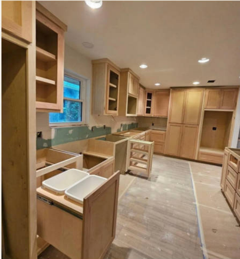
Large kitchen layout in active installation.
